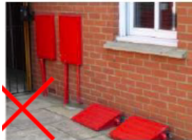
Visible service boxes
