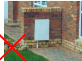
Visible service boxes
